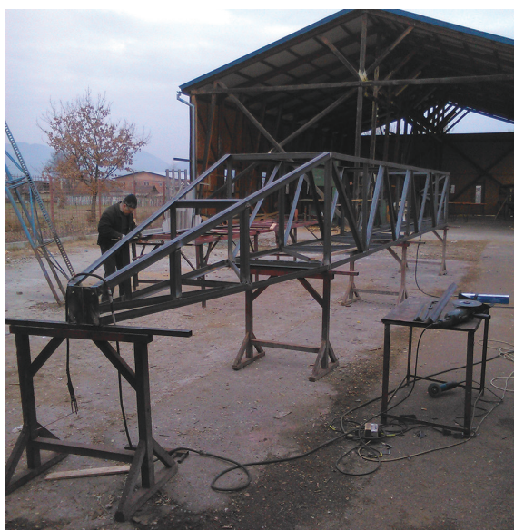
'Undercurrent' under construction
