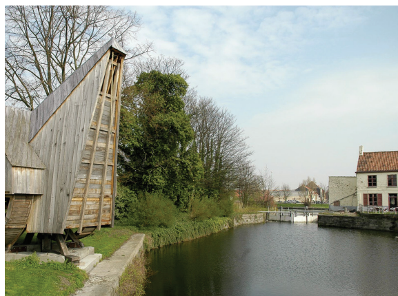
Sasplein with wooden crane
